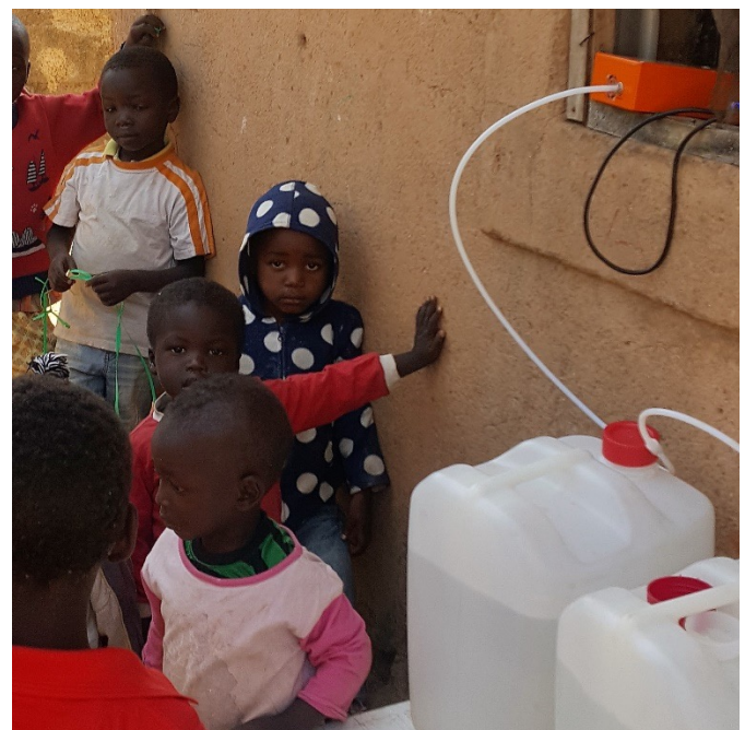
Fig. 2 A small drinking water facility in northern Nigeria, representative of multiple similar facilities in the same region. Ozone is generated by microplasma units, one of which is visible (orange box), and powered by small solar panels (not shown). Each of the microplasma generators is robust and easily repaired in the field with "snap-in" replacement parts.
