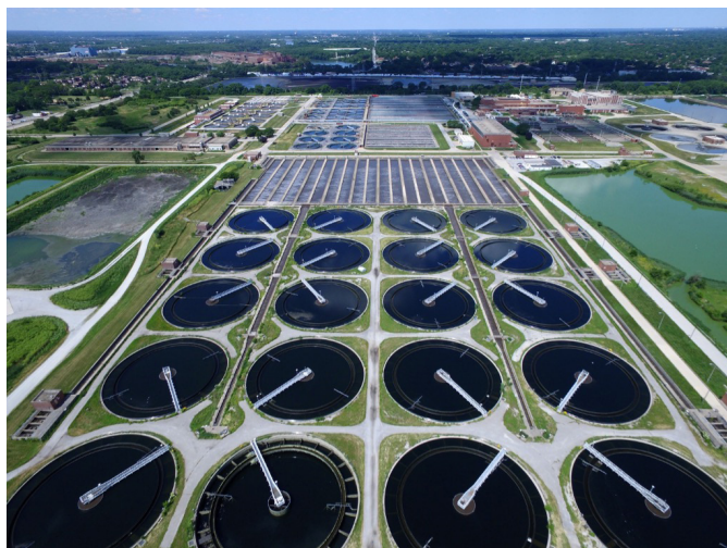
Figure 2. City of Chicago wastewater treatment plant aerial view—processes 700 million to 1.4 billion gallons per day.
